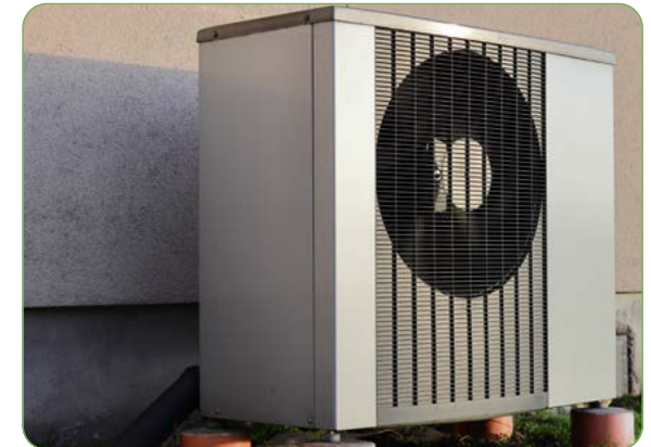
Air Source Heat Pump
