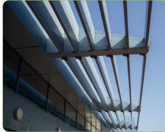
South facing facade incorporating horizontal Brise Soleil
