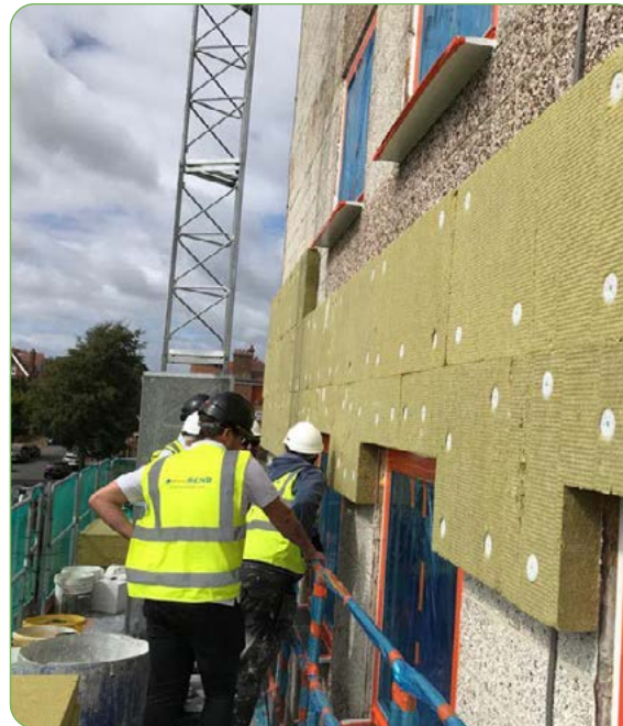
Baumit wall insulation being applied to a multi-residential building. External wall insulation is well suited to old single-brick buildings, being an effective way of treating condensation when insulation is required on one or two walls (source: www.selfbuildanddesign.com )
