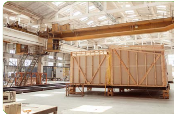
Composite wooden sip panels erected in a factory
