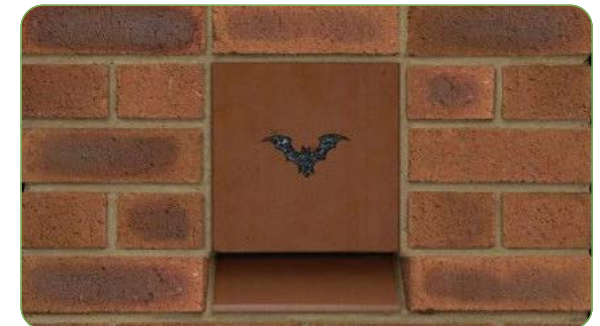
Bat Box built into a wall
