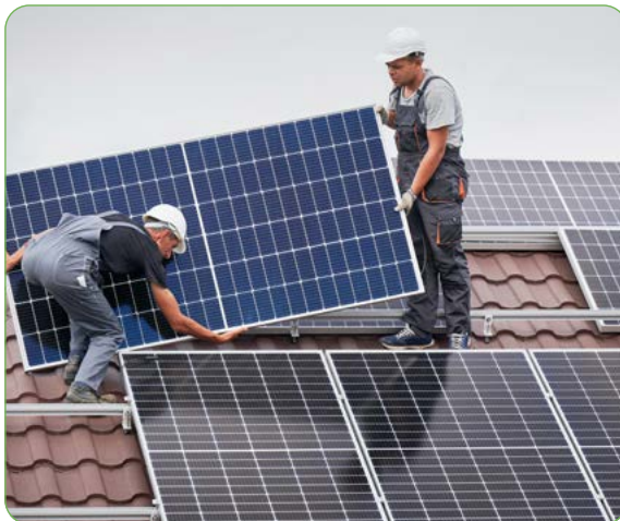
Technicians installing photovoltaic solar modules on the roof of a house
