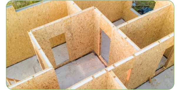
Construction of new and modern modular house. Walls made from composite wooden sip panels with styrofoam insulation inside
