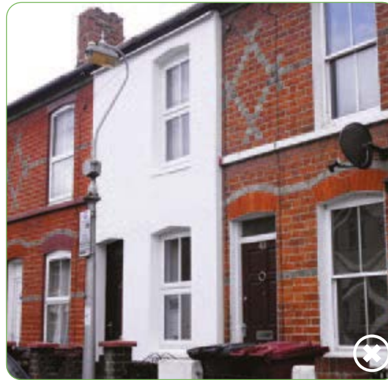
An insensitive external wall insulation application which damages the beauty and character of the street (Source: Planning Responsible Retrofit of Traditional Buildings - Sustainable Traditional buildings Alliance )
