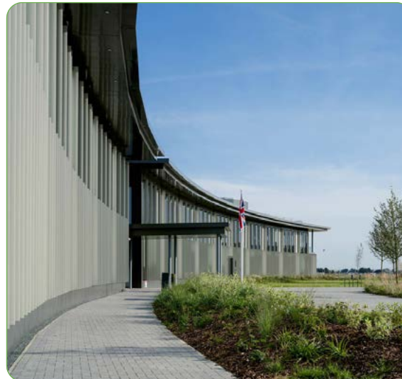
East facing facade incorporating vertical Brise Soleil - New Shire Hall, Alconbury Weald
